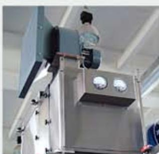
Sterile air filtration system for the air entering the working zones
